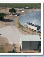
The City pumps water from the Ogallala aquifer and disinfects it near the well field. Then the water flows to Lubbock and enters into the distribution system in Northwest Lubbock.
