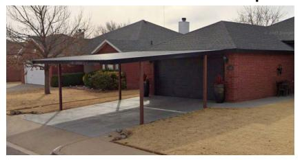
THIS CARPORT WOULD NOT BE PERMITTED. IT DOES NOT MATCH THE ROOF SLOPE, ARCHITECTURAL FEATURES, OR MATERIALS OF THE HOUSE.
